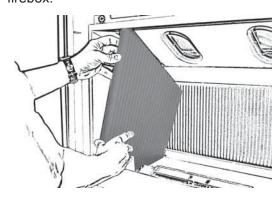
3. Hold the right hand side panel at an angle and insert its bottom edge inside the firebox. Rotate the panel to a vertical position ensuring that the top edge is behind the flange of the firebox. Pull the panel as forward as possible against the right edge of the firebox.
